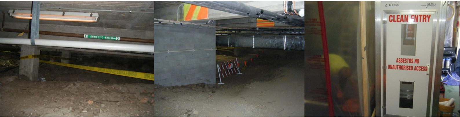
Figure 3.6 – Restricted access to the plant room and undercroft area
