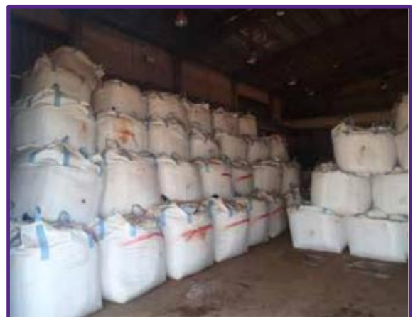
Figure 2.7 – Asbestos stored in bags prior to disposal
