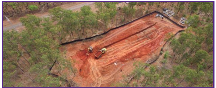
Figure 2.5 – Rehabilitation of a tip site
