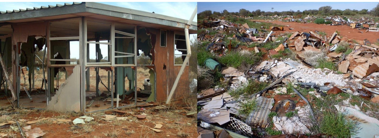
Figure 5.3 – Typical condition of the landfill sites at the start of the program
