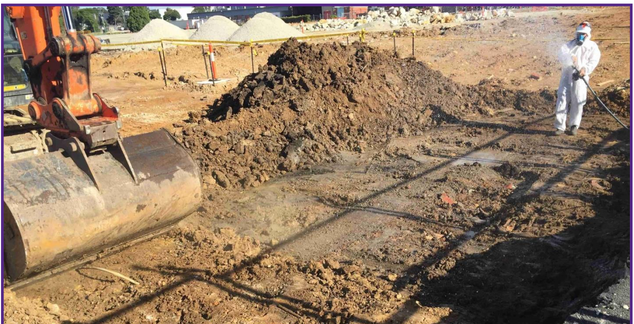
Figure 7.3: Asbestos removalist keeping the asbestos contaminated soil moist
