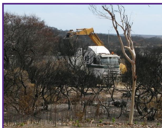
Figure 6.3: Asbestos contaminated materials being loaded into a truck
