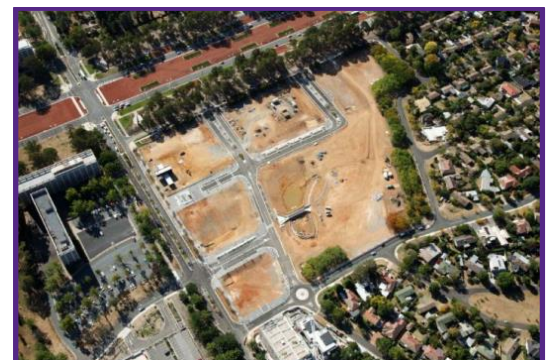
Figure 1.5: Completed site and completed surface works prior to selling the development
