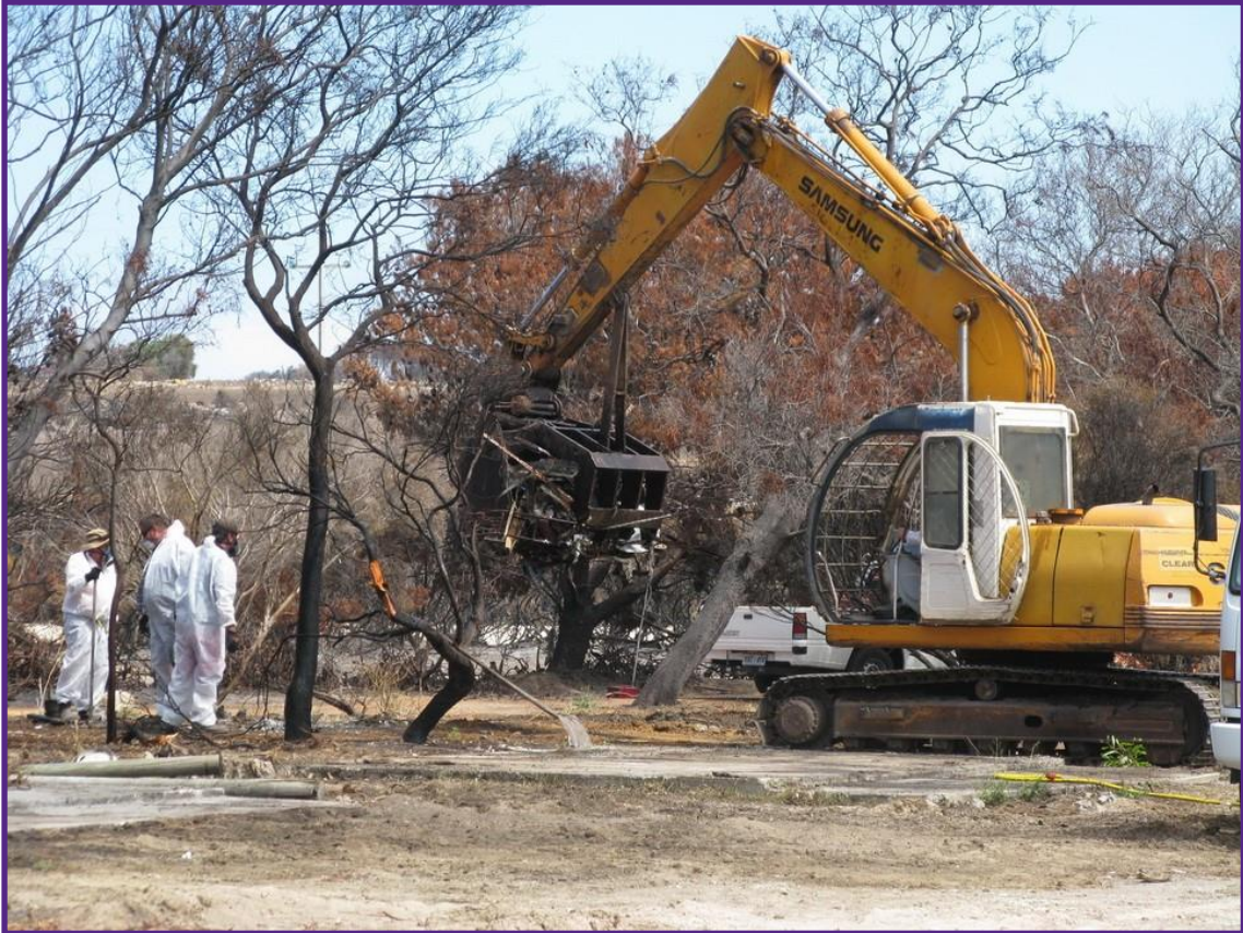
Figure 6.2: Removal of asbestos containing materials
