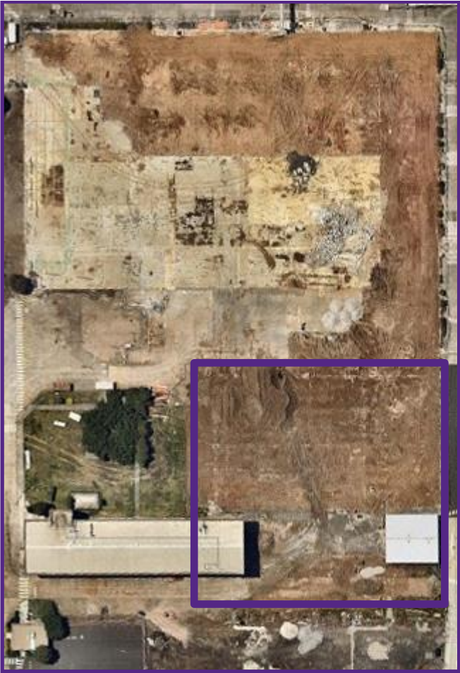
Figure 7.2: A section of the company’s site, with ACM contaminated soil fill area located within the purple square
