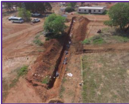
Figure 2.4 – Removal of buried asbestos conduit
