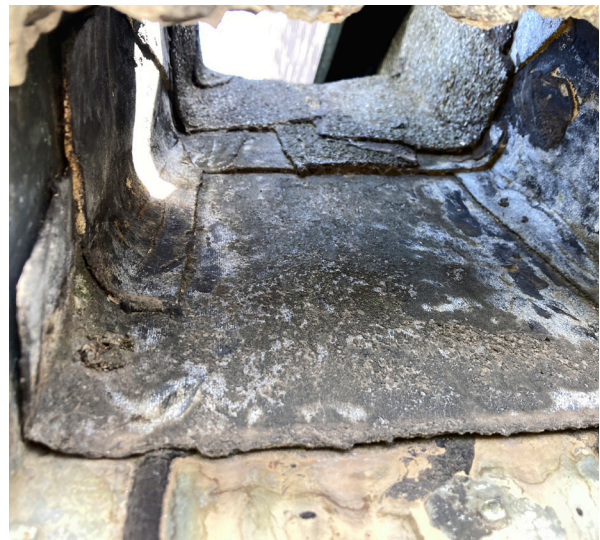
FIGURE 11: Bituminous membrane in water channel
