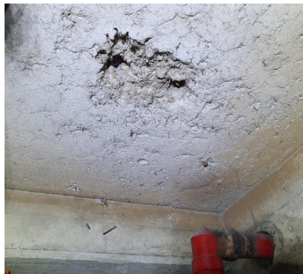
FIGURE 17: Damaged sprayed coating which was originally tamped
