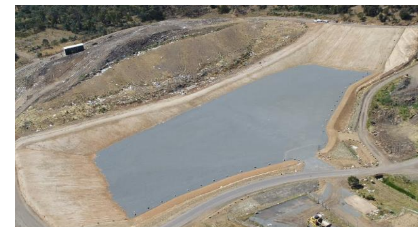
Launceston Waste Centre and Transfer Station, Tasmania
