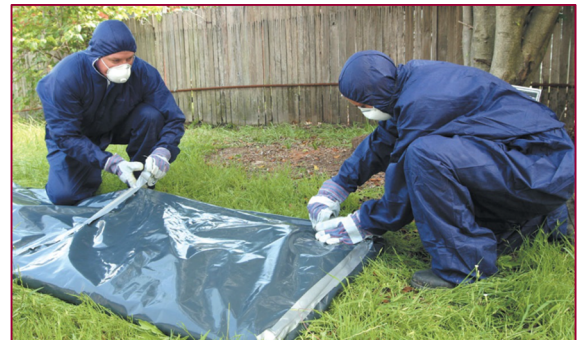
Wrapped asbestos sheeting (Tweed Shire Council)
