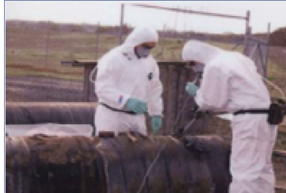
Photos: AC pipe removalists undertaking removal works.
