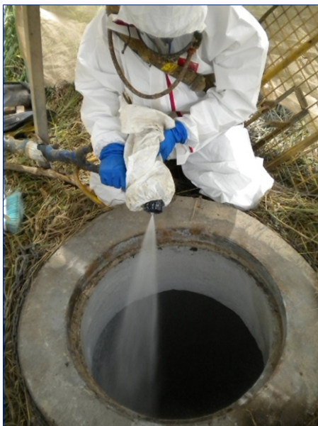
Photo: Manholes, showing signs of deterioration, being repaired. A special coating is applied to restore them to original condition.
