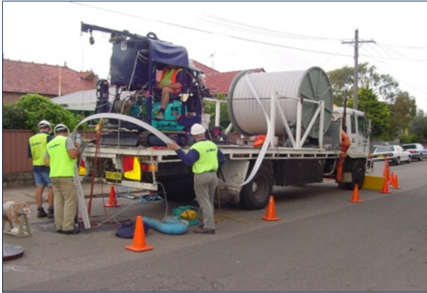
Photo: AC pipes being repaired via trenchless technology.
