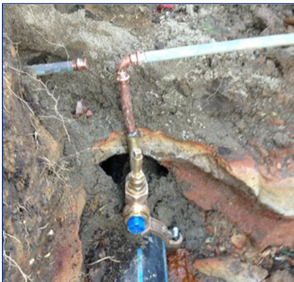
Photos above: The worksite where Shoalhaven Water removed an AC pipe and replaced it with a new water main.
