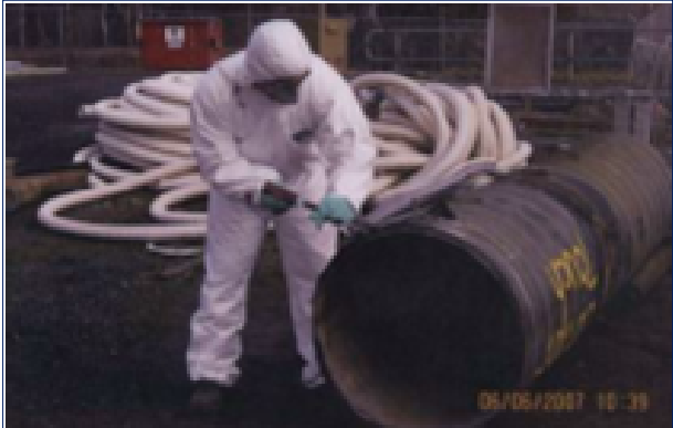
Photos: AC pipe removalists undertaking removal works.
