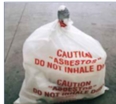
Photo: AC disposal bag, goose necked and sealed.
