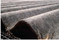
**NON-FRIABLE:** bonded securely as part of another compound, often cement. Can be found as part of cement pipes or fibro sheets. It can be hazardous when disturbed, damaged or deteriorating as asbestos fibres can be released.
