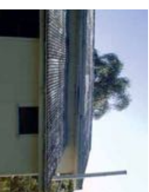
Figure 22: ACM corrugated roofing
