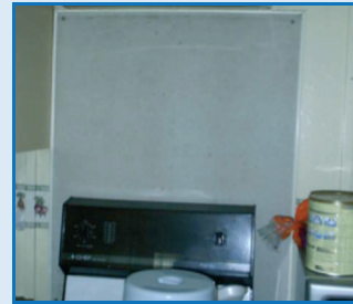
Cement wall linings ...
