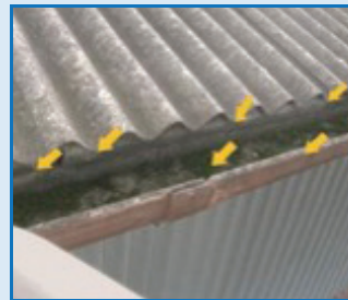
Roofing and guttering
