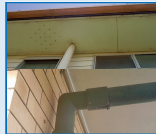
Eaves and downpipes
