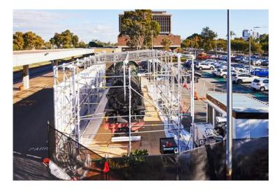
The enclosure was then put under negative pressure. This was to ensure it was completely sealed, so that all particles in the removal area could be sucked out through the filtration system. Thuroona used a manometer to consistently monitor the air pressure throughout the removal process, to ensure there were no leakages. A three door airlock prevented any air movement between the work area and outside.
