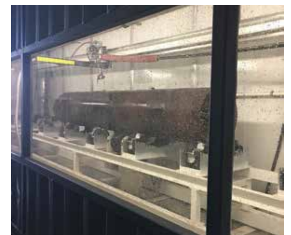
Figure 26: The treatment plant removes personnel manual labour and utilises water pressure to remove the coating from the pipes, supporting pipe reuse or recycling and diverting waste from landfill.
