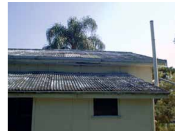
Figure 23: Narrow corrugated AC roof cladding
