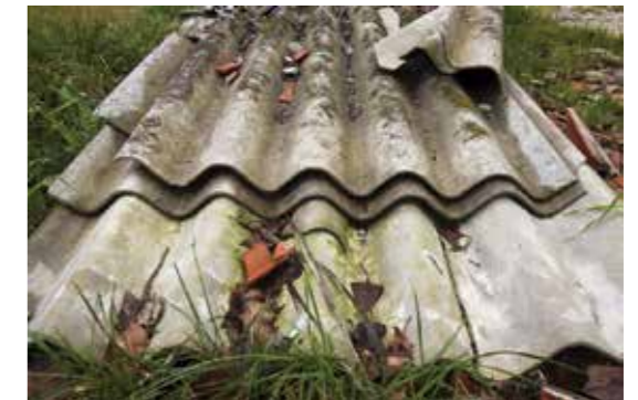
Figure 22: ACM corrugated roofing
