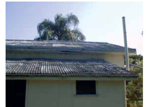
Figure 23: Narrow corrugated AC roof cladding
