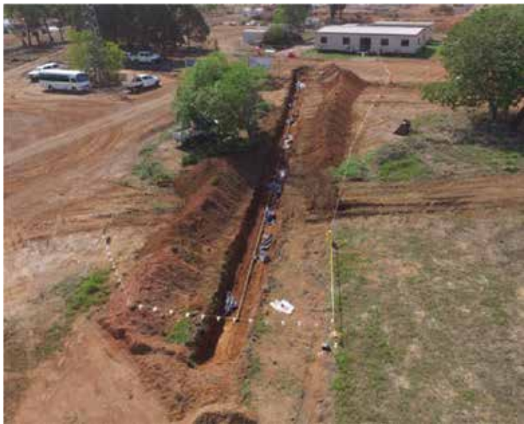
Figure 16: Removal of buried asbestos conduit
