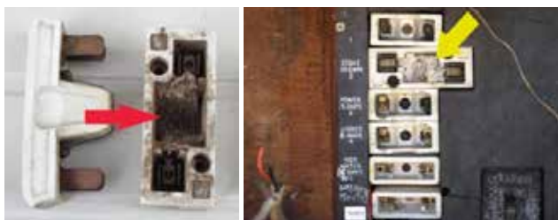
Figure 3: Woven asbestos textile fuse linings are common for large and small fuses.
