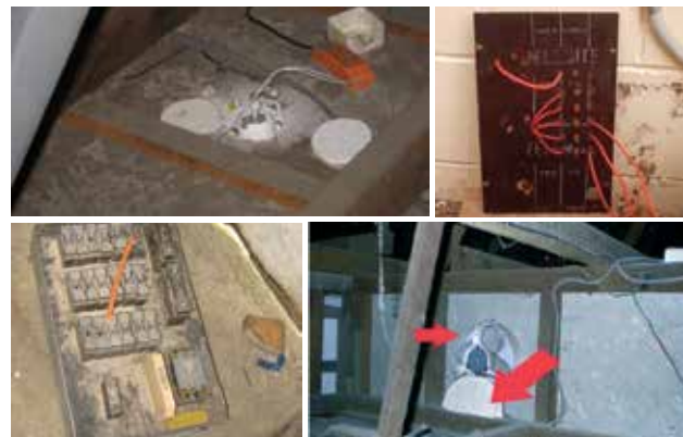
Figure 6: Discarded asbestos waste onsite. Often you will find asbestos debris discarded such as this asbestos insulation board ceiling pieces left lying in the roof, discarded electrical backing board, entire fuse box and asbestos cement pieces where a ceiling extractor has been installed.
