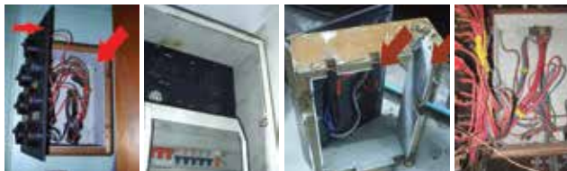
Figure 2: Asbestos cement and asbestos insulation mixed linings inside the electrical box itself.
