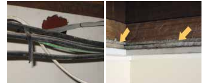
Figure 7: Take appropriate safety precautions including P.P.E. when running cables through asbestos and do not leave an asbestos mess for next time. The ongoing renovation boom in Australia has resulted in asbestos-containing materials being hidden to be found later by another tradesperson.
