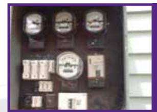
Electrical meter backing boards
