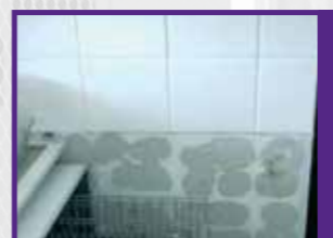
Asbestos lining behind tiles
