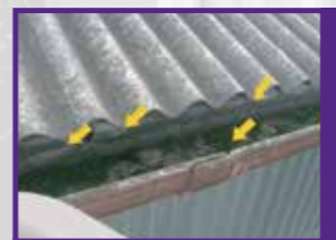
Cement roofing, and gutters
