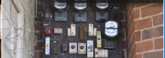
Electrical meter boards
