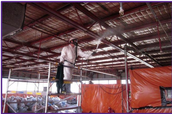
Figure 1.4: Asbestos removal in progress
