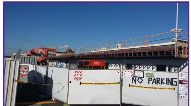
Figure 3.4: Exclusion zones set up around the site
