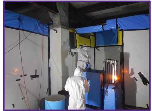
Figure 4.5 Asbestos removal works were undertaken in enclosed areas
