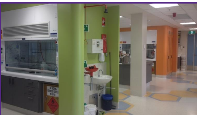
Figure 7.8 – Example of the new laboratories
