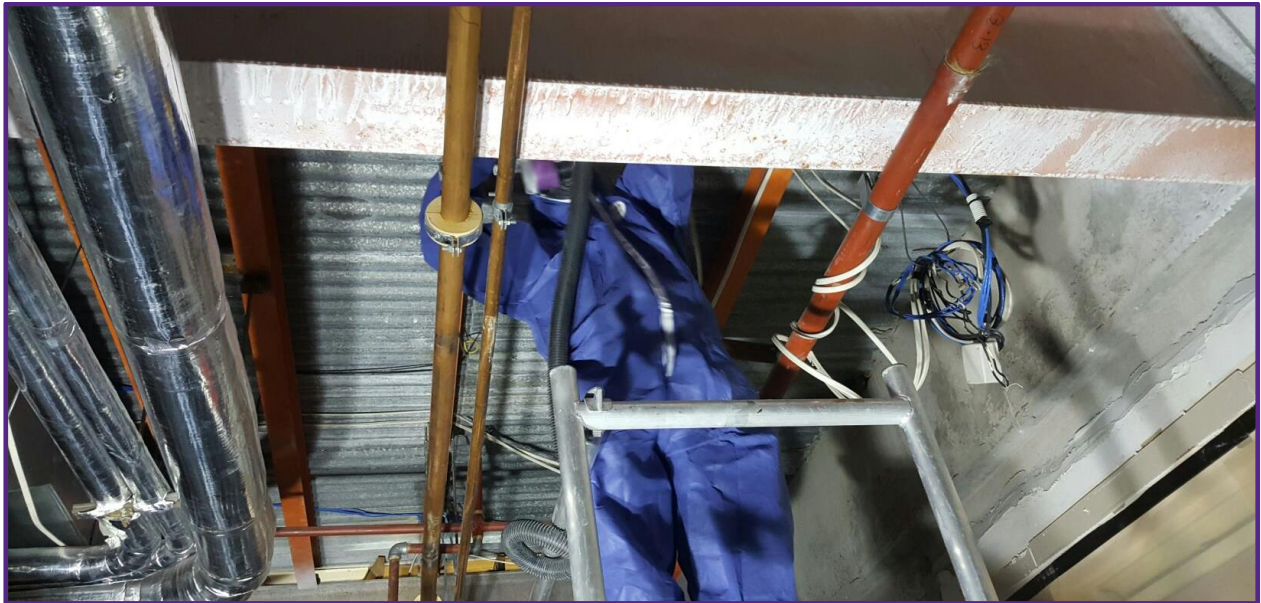
Figure 5.5: Asbestos removalist treating a beam in the ceiling
