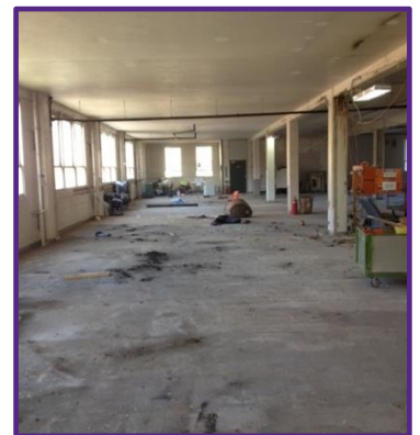
Figure 7.7: Area after demolition
