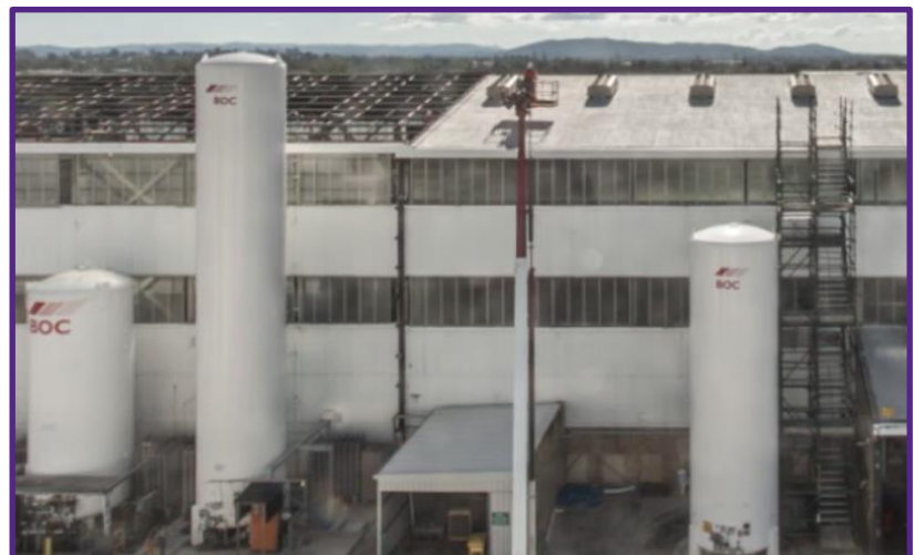
Figure 3.5: Removal of asbestos sheeting from warehouse
