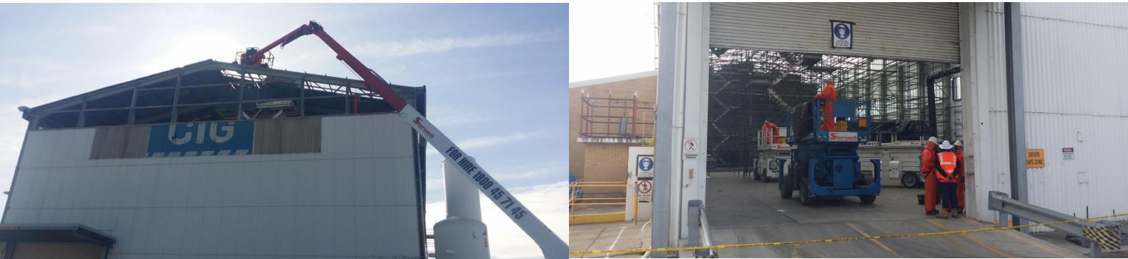
Figure 3.7 – Removal of Asbestos roofing (left image), contractors on site (right image)
