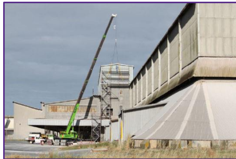
Figure 11.2: Crane and scaffold access
