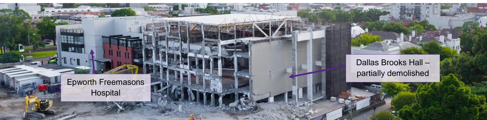
Figure 4.3: location of asbestos removal works in relation to the hospital
