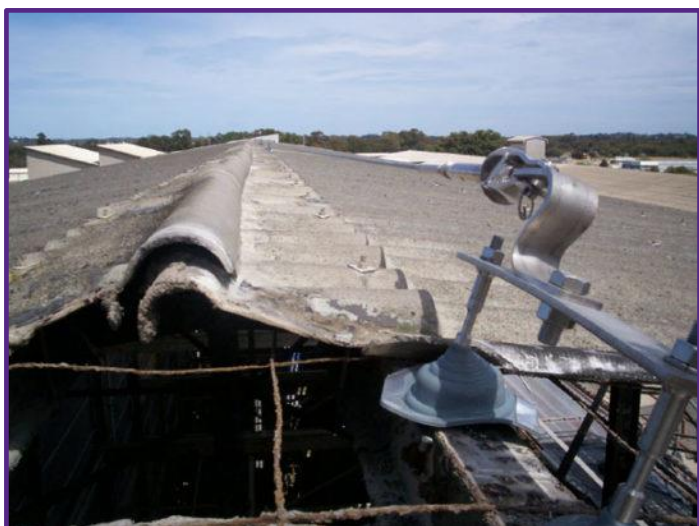
Figure 11.4: Asbestos roof sheeting on warehouse
