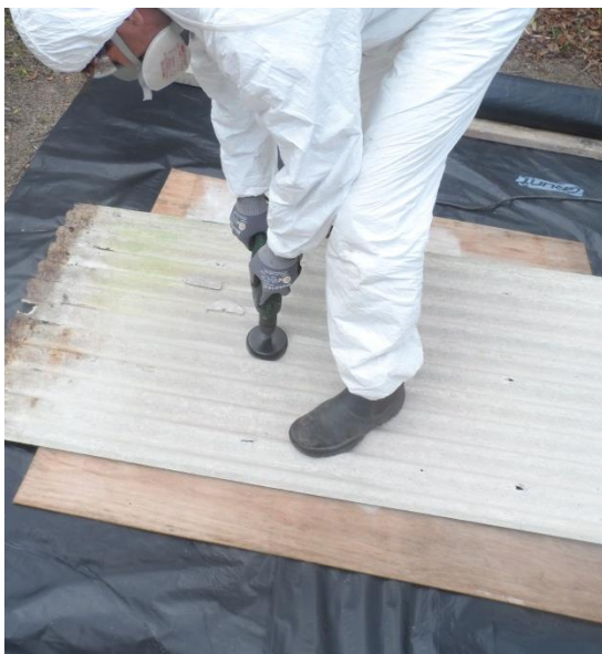
Figure 3 Flue Penetration in AC Sheeting
