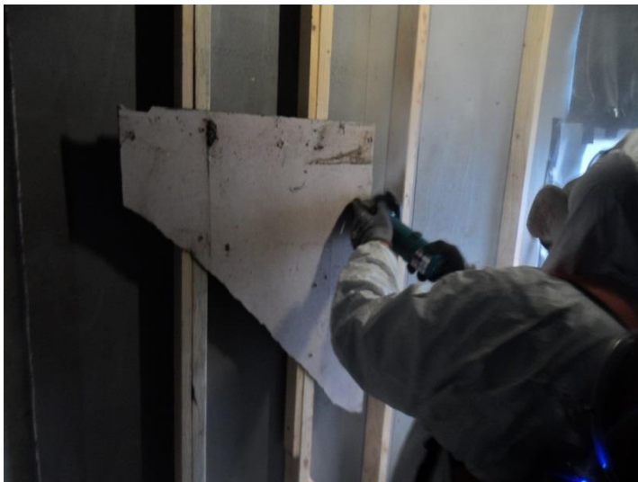
Figure 4- Cutting AC sheeting
