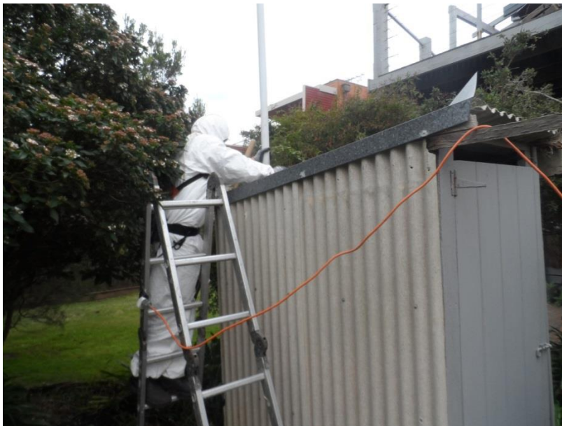
Figure 5- Removal of Asbestos Sheetting from small shed
